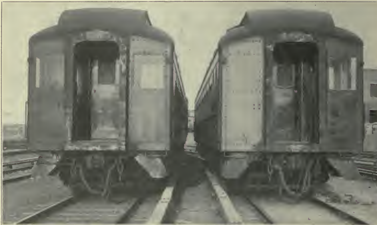
FIG. 511. YARD TRACK CONSTRUCTION, 600-VOLT OVER RUNNING THIRD RAIL Position of Passenger Coaches with Reference to Third Rail, Sunnyside Yard, Pennsylvania Railroad, Long Island City, N. Y.
